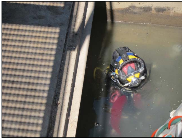
Seawater Pumping Station cleaning
