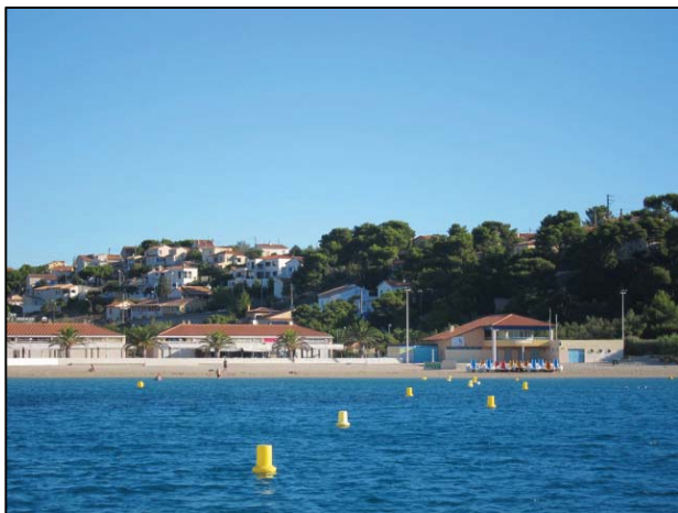
Beach Beacons - Martigues
