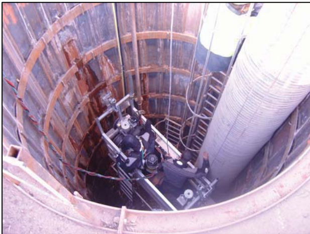
Intervention in a well
